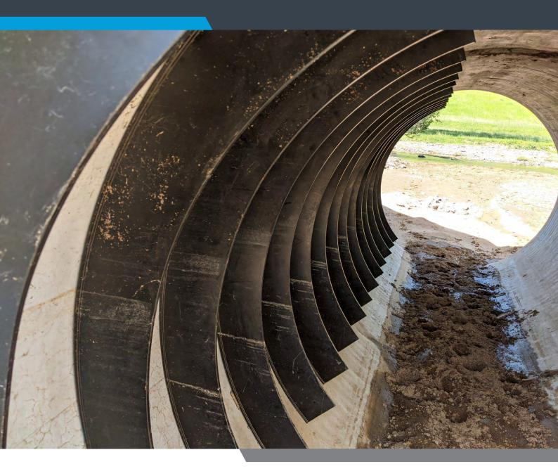
HDPE Fish Baffles are fixed to the pipe's interior to improve the culvert's conditions and assist fish migration. Furthermore, fish can find shelter from predators between the baffles during low flow, as small pools of standing water are formed. HDPE material is used to customise any size or shape, along with its high resistance and durability to weather and impact over time.
