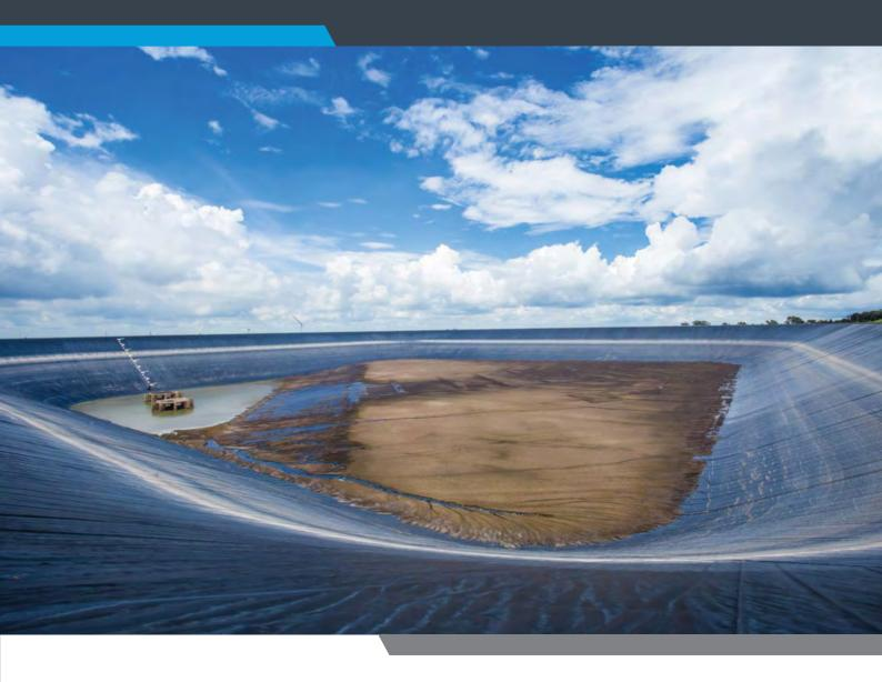
HDPE Pond Liners (Geomembranes) are used to create waterproof impermeable barriers. The installation process involves rolling out large, pre-defined, HDPE Liner (Geomembrane) sheets and welding the edges. In doing so you create an impermeable barrier that will keep the given media from leaking into the surrounding environment. We also offer Liner Lite for smaller projects.
