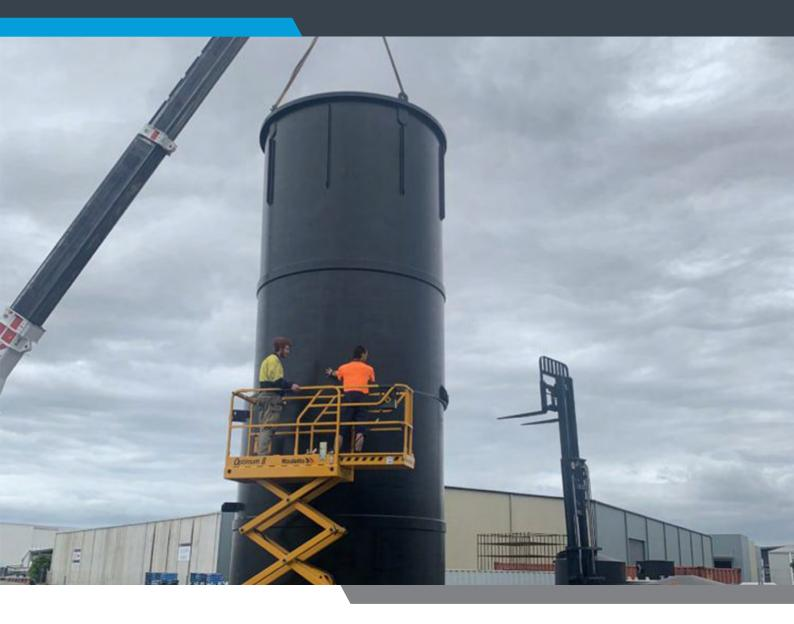
A self-bunded tank is a storage tank that has an inner and outer tank with a gap in between. The bunding captures any leakage that may occur from the first tank to ensure the hazardous chemicals are contained. Put simply, it is a tank within a tank and very similar to an IBC Bund but on a much larger scale. These types of tanks are common in any process that requires hazardous materials.
