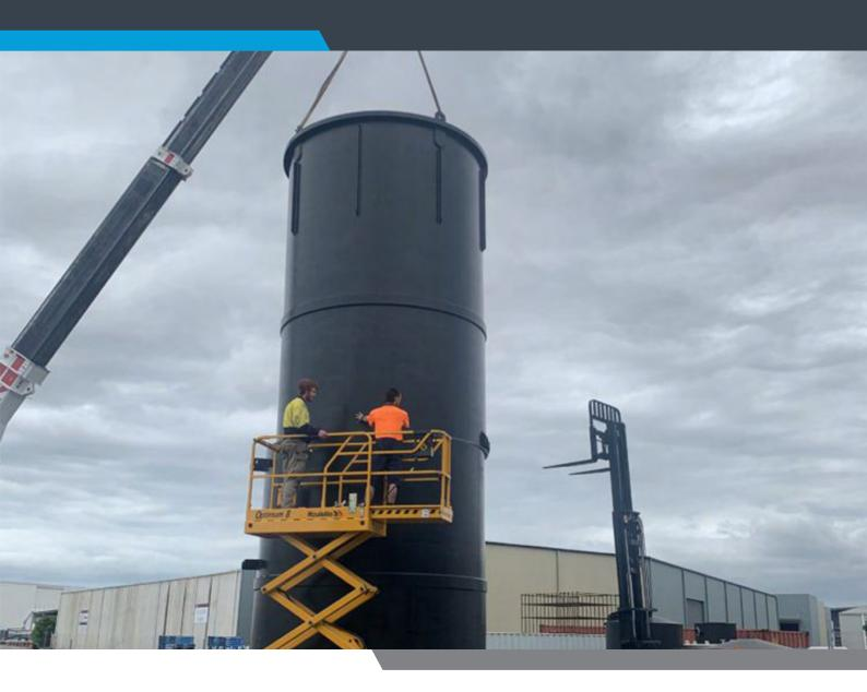
A self-bunded tank is a fuel storage tank that has an inner and outer tank with a gap in between. The bunding captures any leakage that may occur from the first tank to ensure the hazardous chemicals are contained. Put simply, it is a tank within a tank and very similar to an IBC Bund but on a much larger scale. These types of tanks are common in any process that requires hazardous materials.
