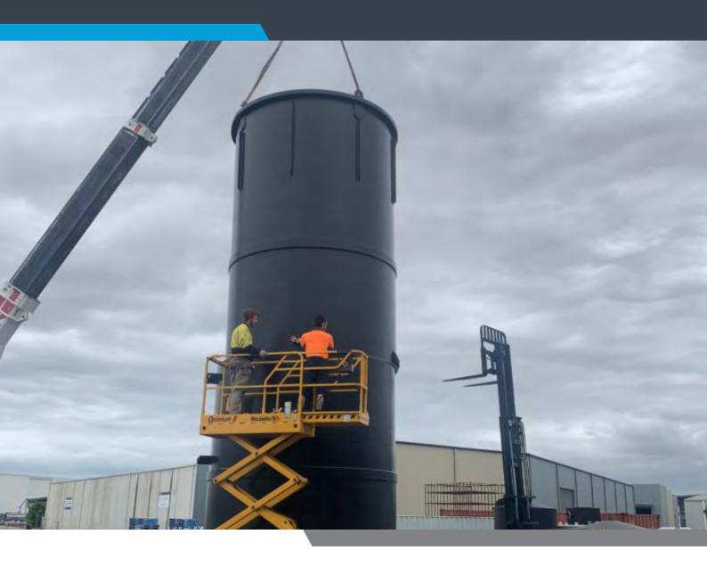
A self-bunded tank is a fuel storage tank that has an inner and outer tank with a gap in between. The bunding captures any leakage that may occur from the first tank to ensure the hazardous chemicals are contained. Put simply, it is a tank within a tank and very similar to an IBC Bund but on a much larger scale. These types of tanks are common in any process that requires hazardous materials.
