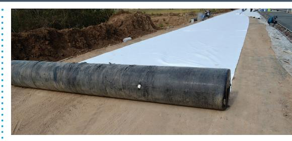
Industrial Plastics offer Geotextile as an option for ground stabilisation, soil bed reinforcement, filtration, erosion control and slope protection. The thinner textiles are manufactured by interlocking fibers while the thicker Geotextile is made from chemically bonded textiles.
